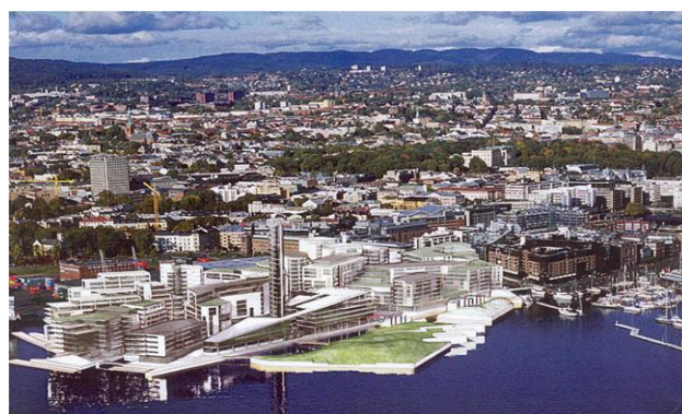
Fig. 1. A new city development currently under construction in the harbor region of Oslo City [17]
